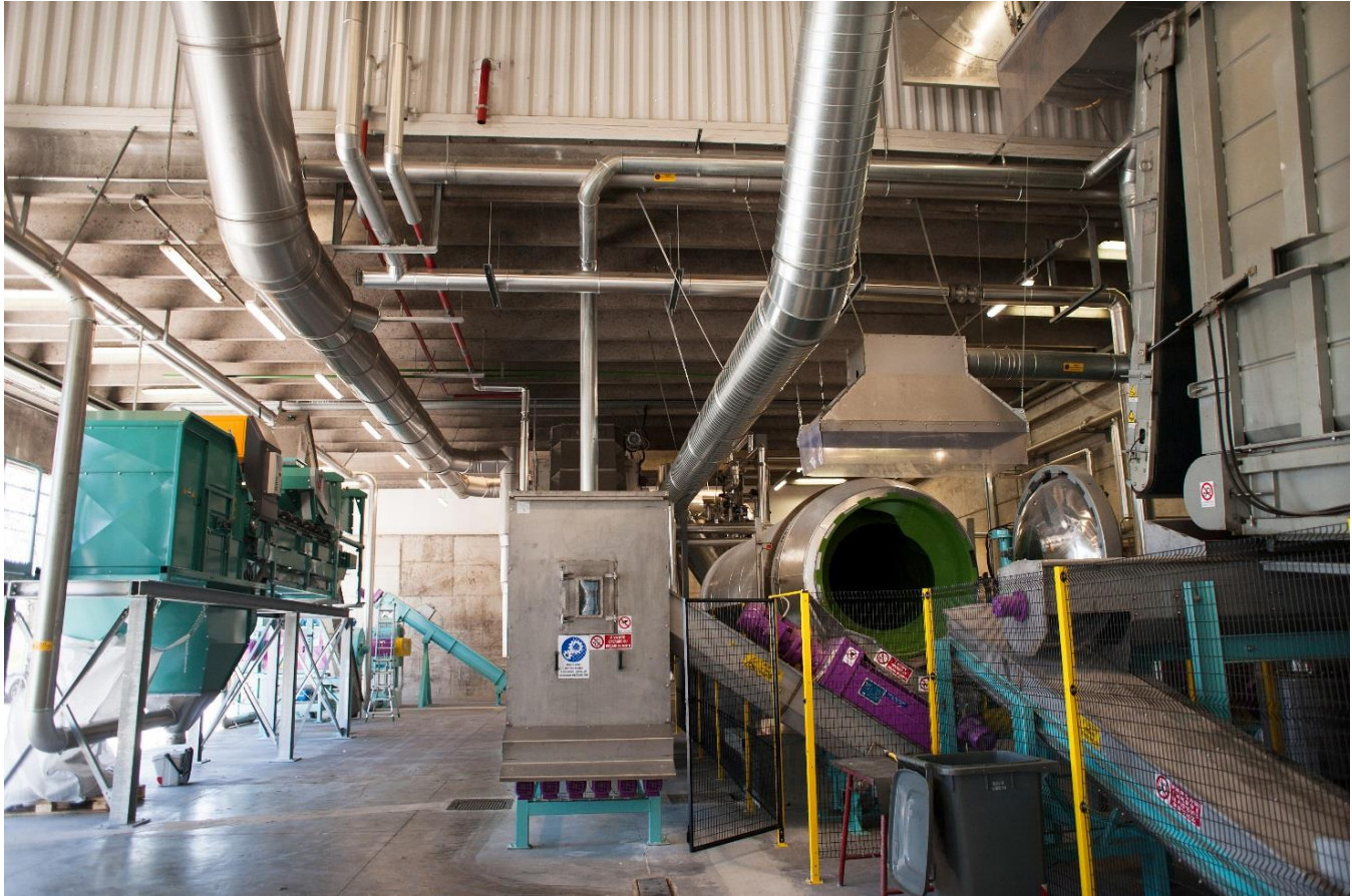
AHP waste pre-treatment plant
